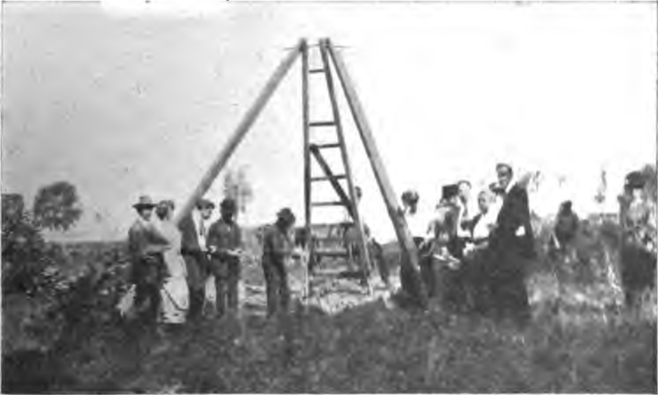
BEGINNING FIRST BORING—FRIENDS HOLDING SOIL IN HANDS
